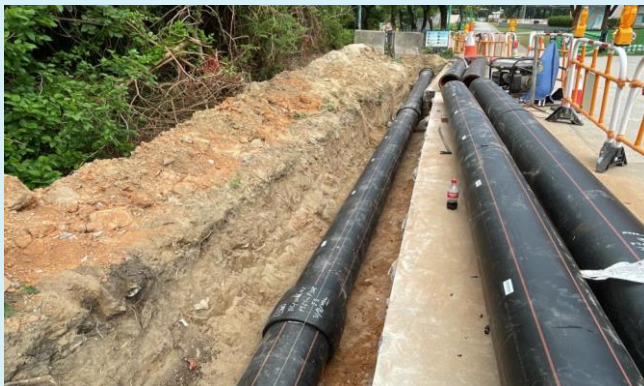
沿貝澳沙灘路鋪設污水管道 Sewer Laying along the Access to Pui O Beach
