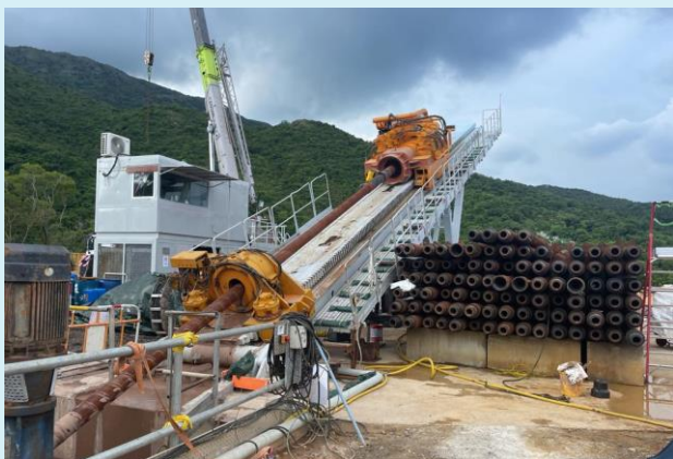
海底排放管道正進行施工 Submarine Outfall Construction in Progress
